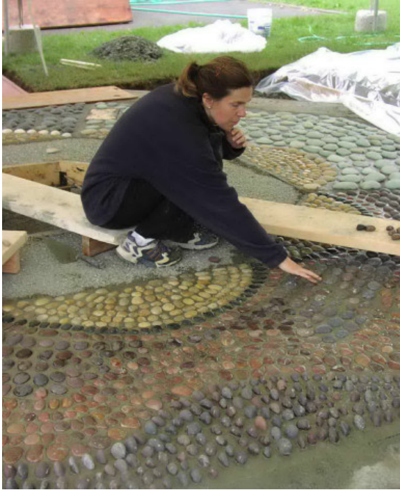
Elizabeth Marazita places stones during construction of the reflexology paths
